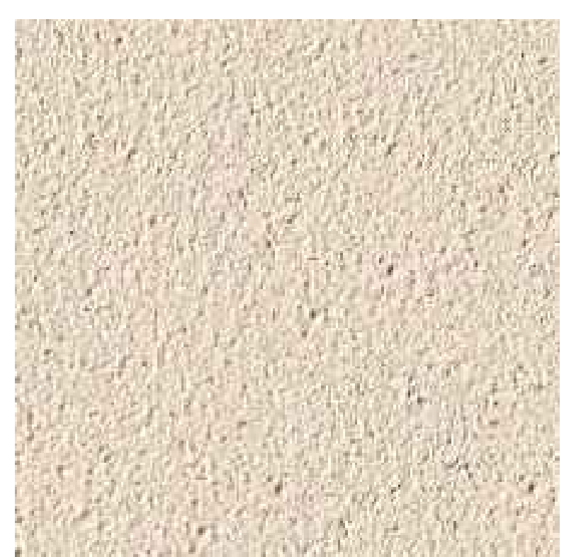
1 EXTERIOR CEMENT PLASTER
